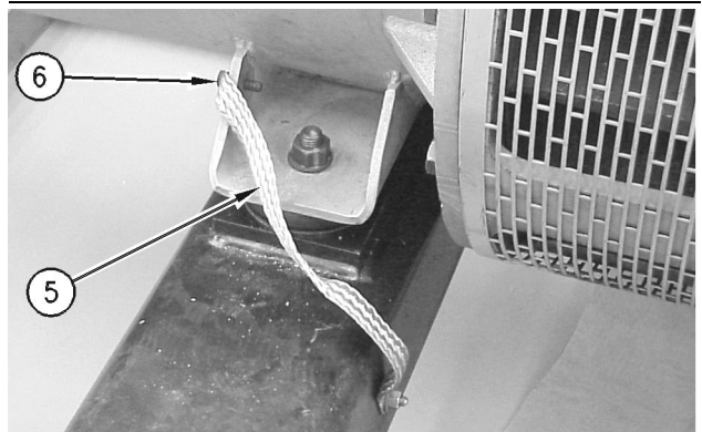
Illustration 92 Generator ground strap (5) Ground strap (6) Bolt
