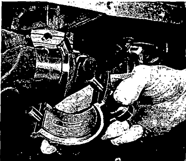
Figure 164—Removing Connecting Rod Cap
