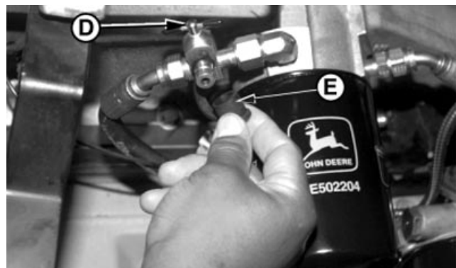
Air Purge Valve
