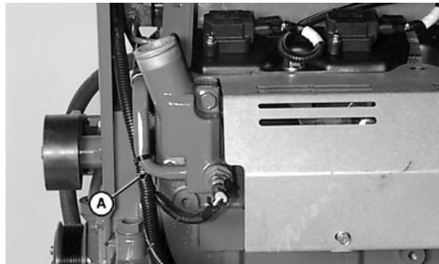
Installing Water Pump Tube
