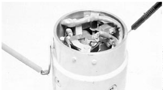
Make Ground Circuit Test
