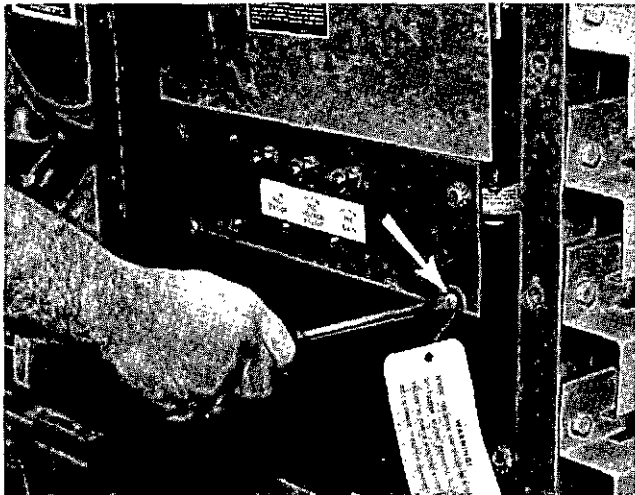
REMOVE SHIPPING SCREWS BEFORE STARTING (SRCR ONLY)
