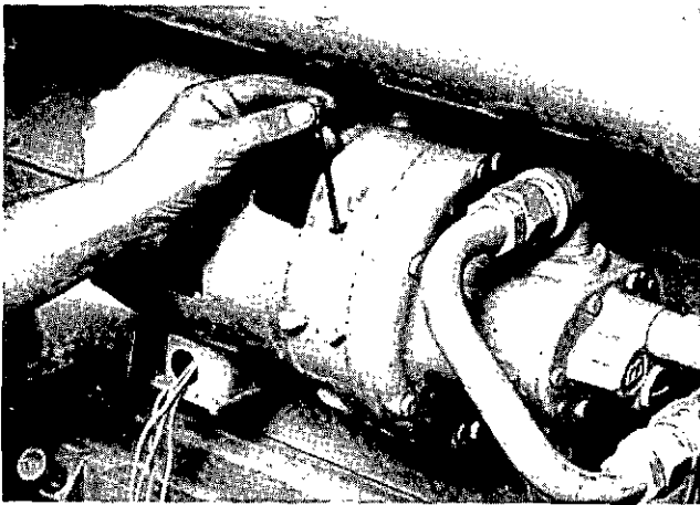
CHECKING OIL LEVEL
