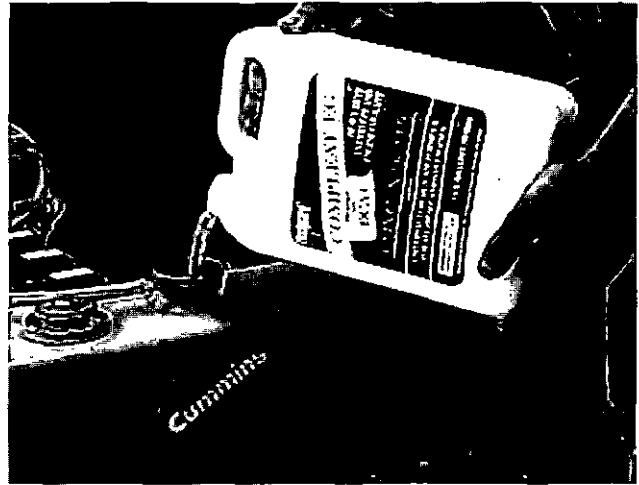
Photo # 7-49 - Filling Cooling System
