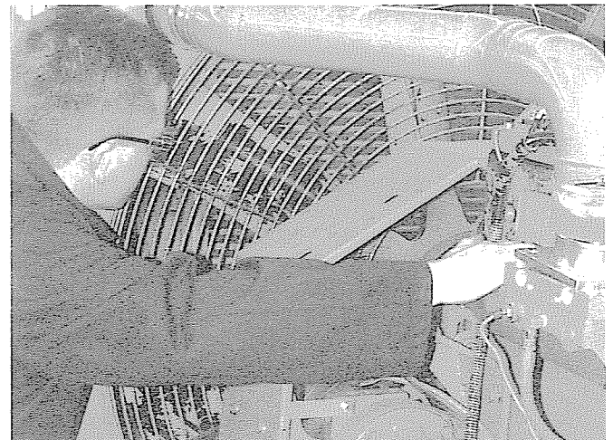
Photo #7-13 - Radiator & CAC (Charge Air Core) External Inspection
