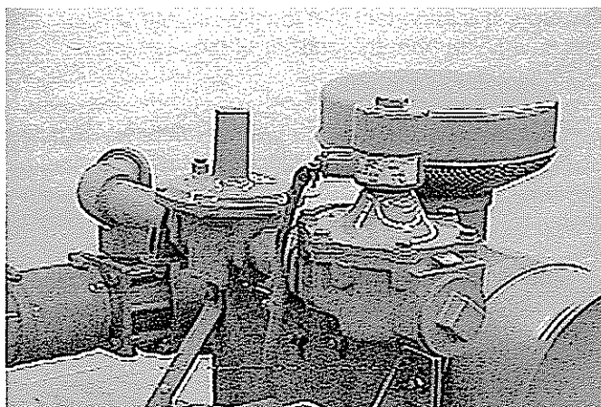
Photo #3-04 - Automatic Gas Shut-Off Valve
