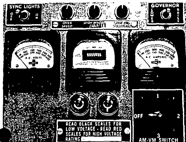
Fig. 2-19, N11825. Typical generator set control panel
