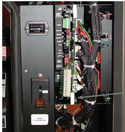
Fig. 7-5, ECM with Connectors Attached
