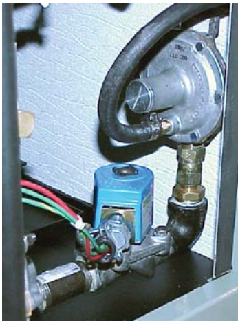
Fig. 7-6, Pre-regulator Removal
