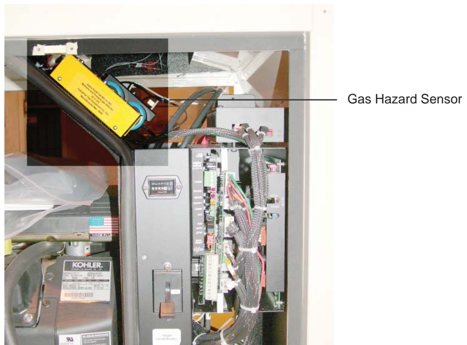
Fig. 7-3, Gas Hazard Sensor Location (Alpha P/N 744-891-20)
