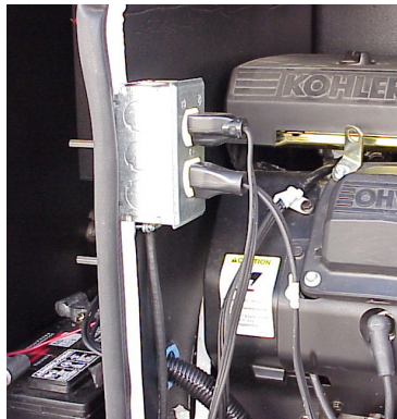
Fig. 7.2 ECM/APU Interconnection (96V Units)
