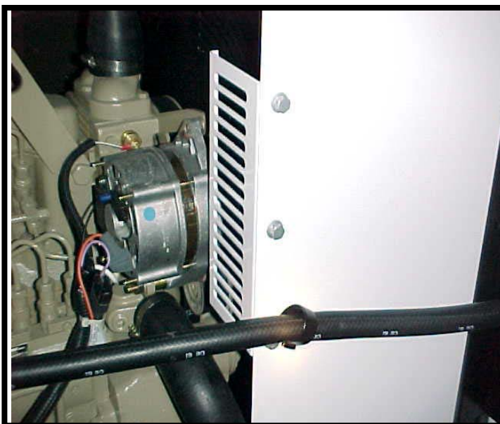
Figure 2 Routing Blow By Hose (Fan Cowling)
