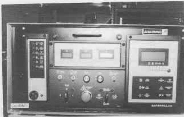
Electronic Modular Control Panel (EMCP)
