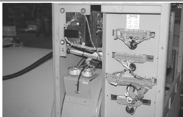
Illustration 85 g00619117 Terminal Strips (DIN)
