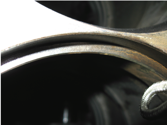
Figure 8. Cracking around counterbore circumference.
