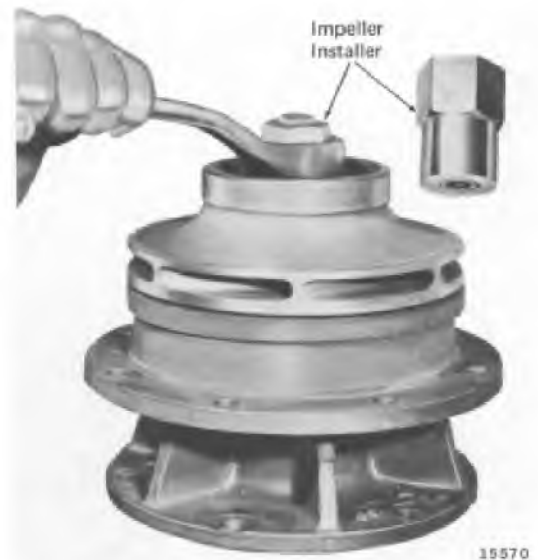
Fig. 10-12 - Installing Pump Impeller
