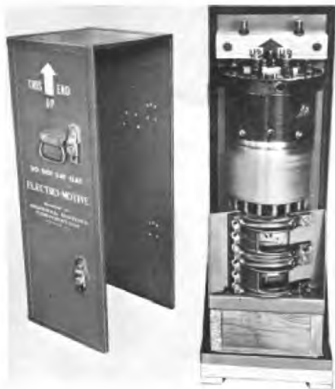
Fig. 5-28 - Power Assembly And Container
