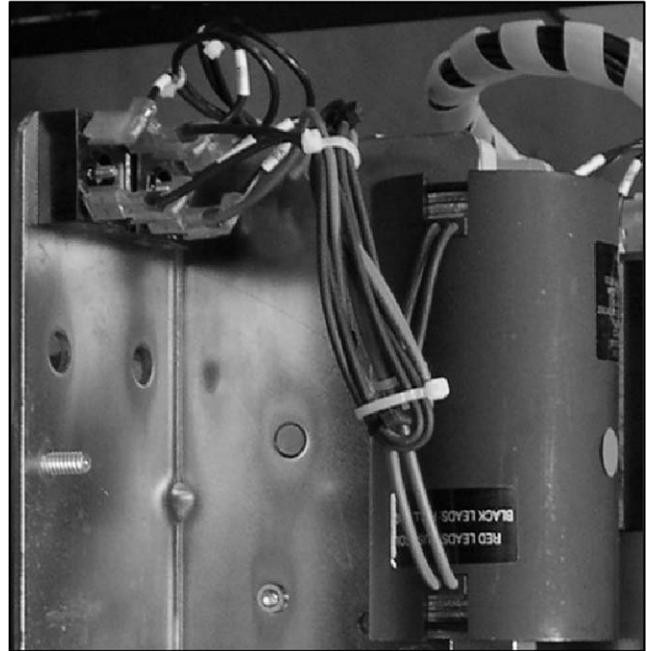
**Figure 5-23** Rectifier Connections and Tie Wraps
