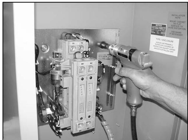
**Figure 5-6** Installing the Power Panel
