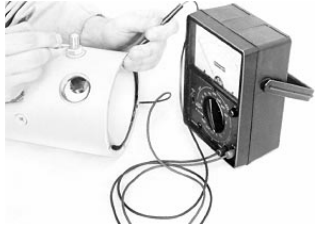
Make Ground Circuit Test
